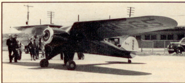
When the Bureau of Air Commerce suggested using low-cost automobile engines to develop an Everyman's airplane, Swen Swanson's coupe design was revamped to include an 80-hp Chrysler/Plymouth engine.
